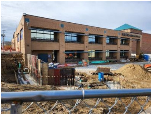
Sojourner Truth Memorial Plaza under construction in Feb. 2023.
